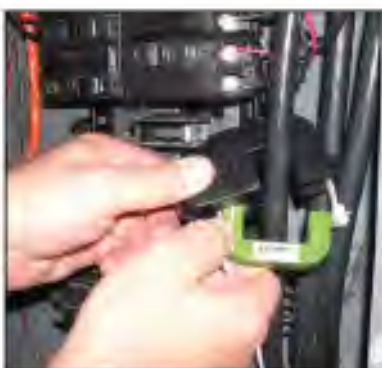
Split-core current sensors install without power interruption in new or retrofit applications.
